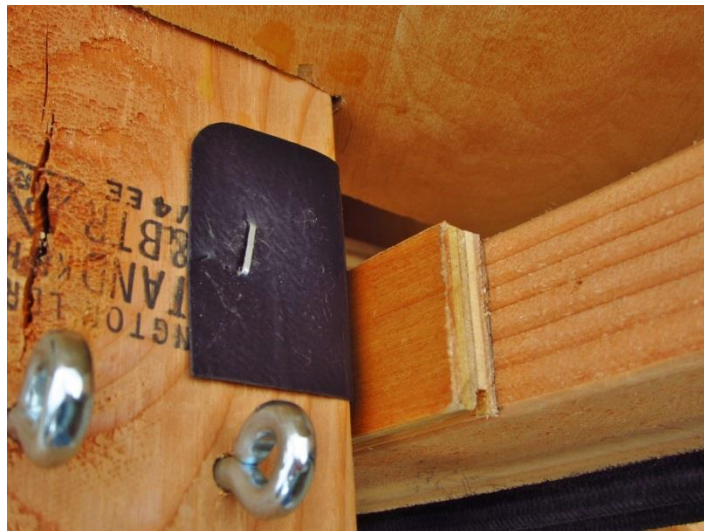
Figure 12: The support slider with anti-stiction binder plastic.
